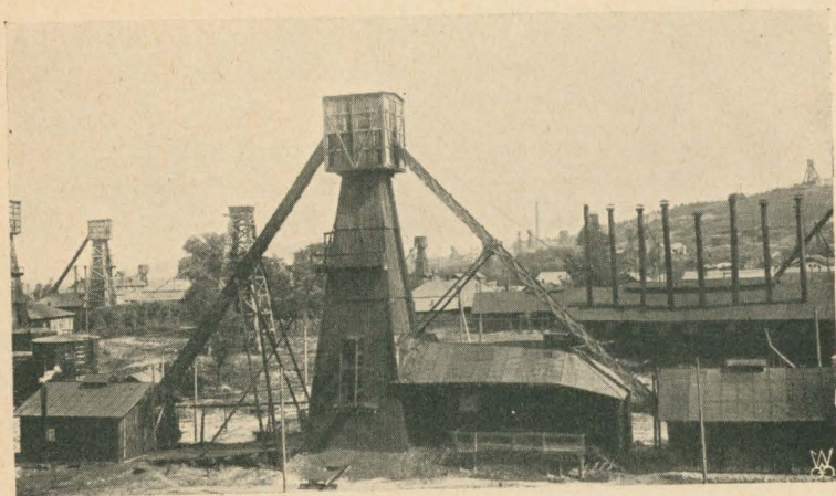
Fig. 1. Canadian rig. Two steam driven hoists for swabbing.
