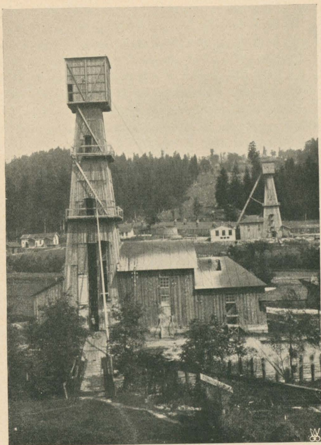
Fig. 4. Combined „Polish“ rope and rod rig with steam drive.
