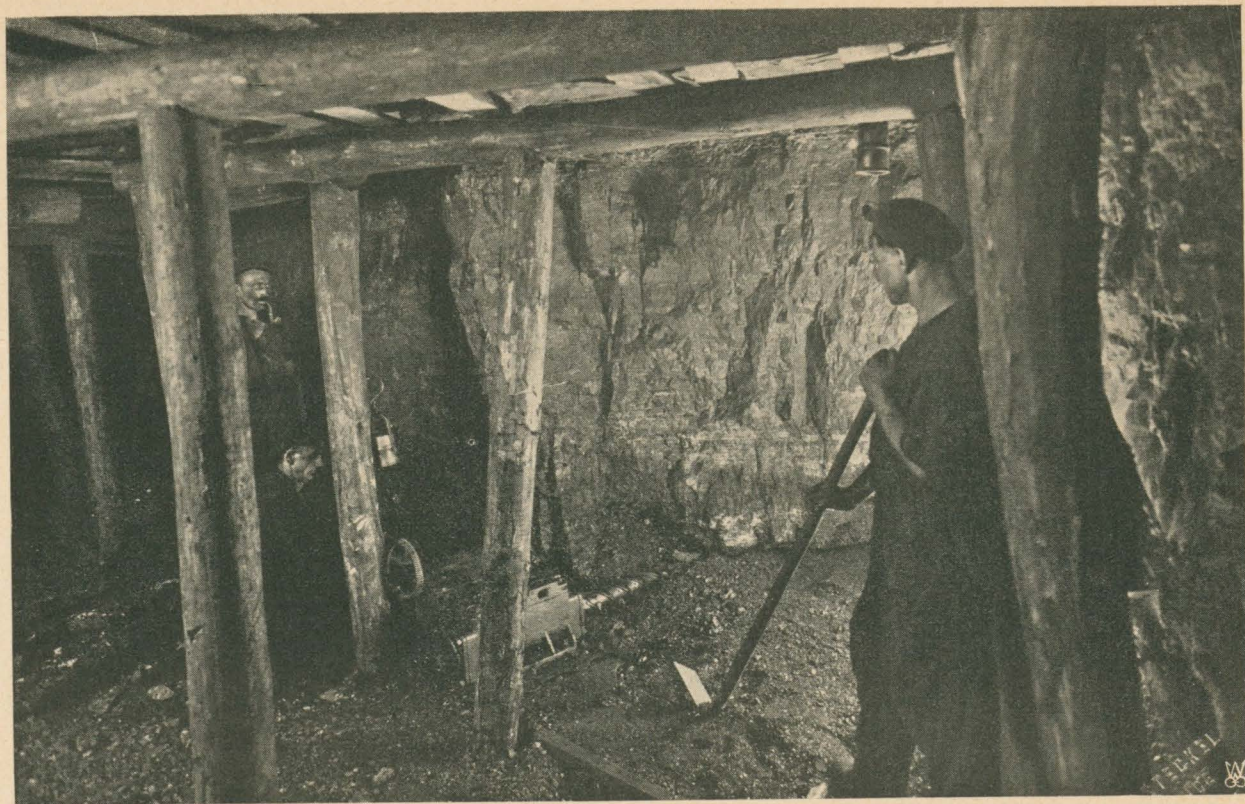
Fig. 3. Breaking out of coal by means of a drilling machine.
