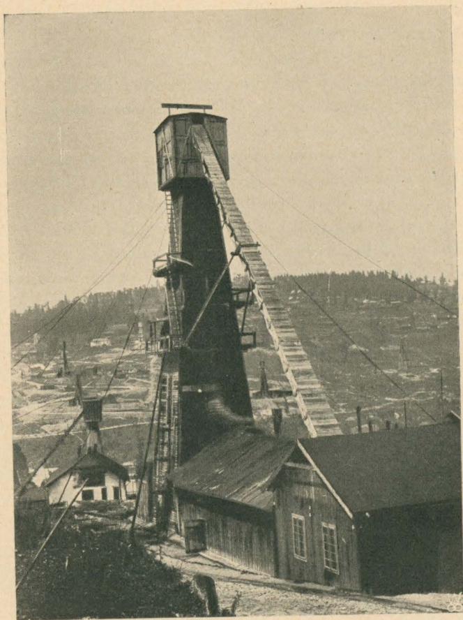
Fig. 5. Combined „Polish“ rope and rod rig. Electrically driven hoist for swabbing.
