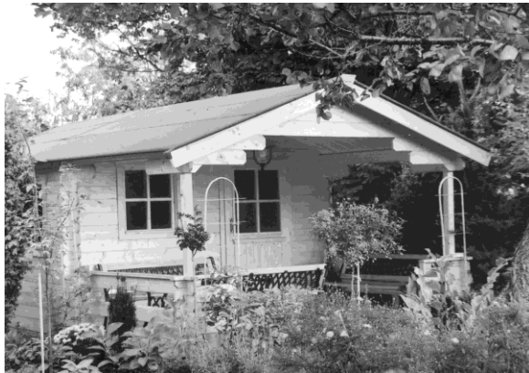
Figure 2. Typical allotment chalet built by a professional company with the use of wooden pre-fabricated units. Allotment sheds come in different sizes and designs, although the local authorities do not regulate their appearance – even though the limit of floor space (30 sq m) has to be strictly obeyed (Anna Pawlikowska-Piechotka 2008)
